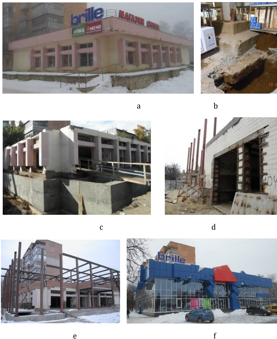
Figure 2. Engineering and geological investigations and some stages of reconstruction of a one-storey building with its extension and superstructure: a - before the reconstruction; b - examination of base and a separate foundation for the column from a pit in the basement; c - excavation of a pit around the existing facility and dismantling of structures; d - reinforcement of concrete frame columns and brick pillars of outside walls; e - installation of columns of extension and second floor, roof beams; f - the building after its extension and superstructure.
