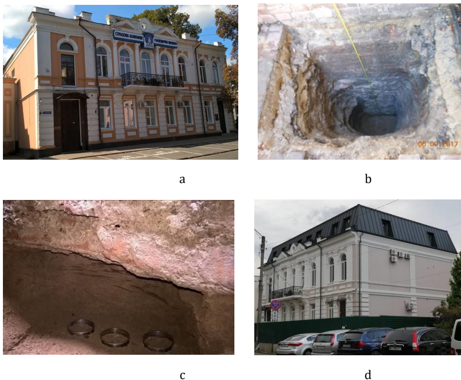
Figure 1. Engineering and geological investigations of a two-storey building with shallow foundations on a natural base: a - building before superstructure; b - pit from which bases and foundations of the building were investigated; c - sampling of rings with long-term compressed soil from under the foundation footing; d - building after its superstructure with an attic floor.
