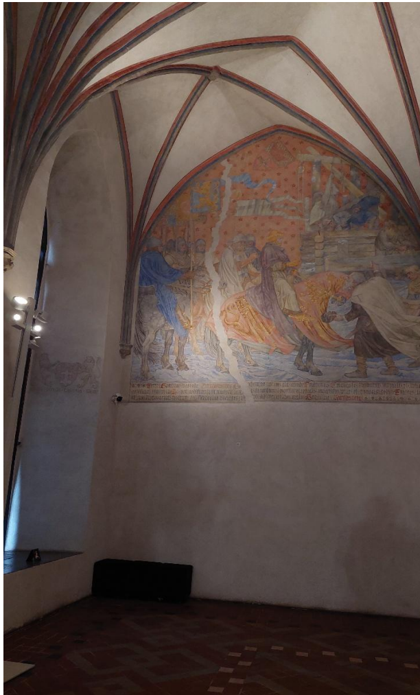
Fig. 4. Elimination of cracks on the premises of the Great Refektarz, 2025
