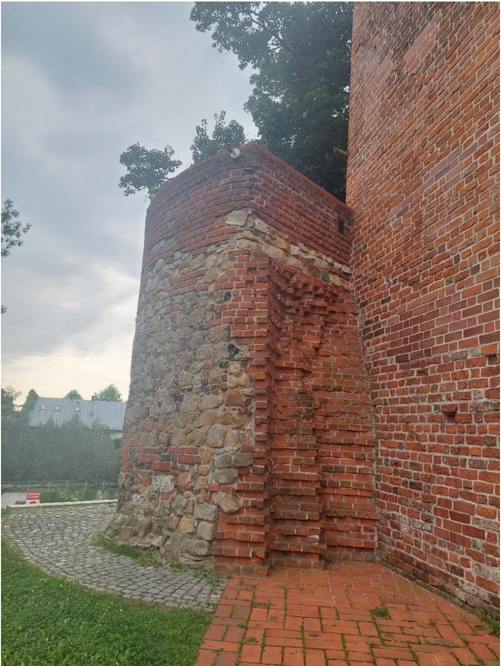
Fig. 6. Fragment of the tower's masonry, 2024
