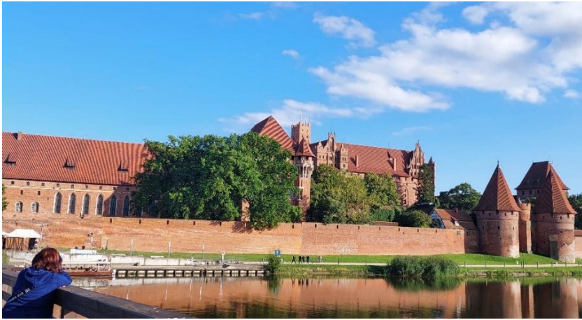
Fig. 8. View of Malbork Castle and the recreation area from the bridge (2025)
