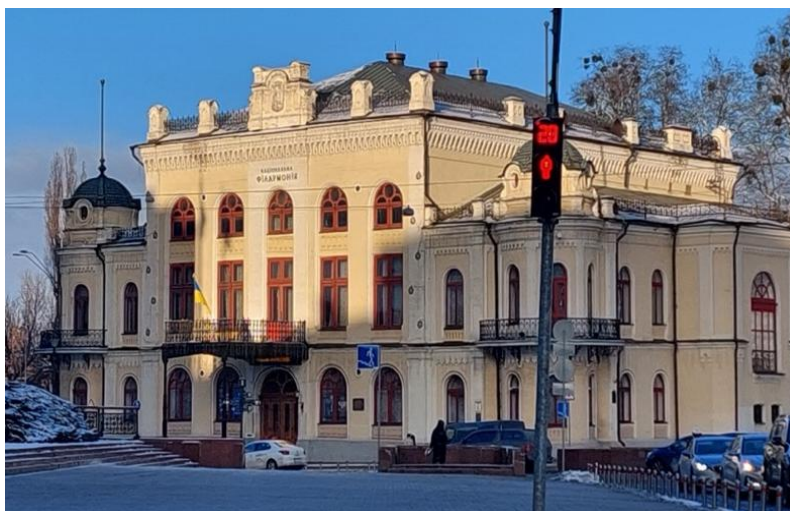
Fig. 5. The building of the National Philharmonic of Ukraine. Modern view.
