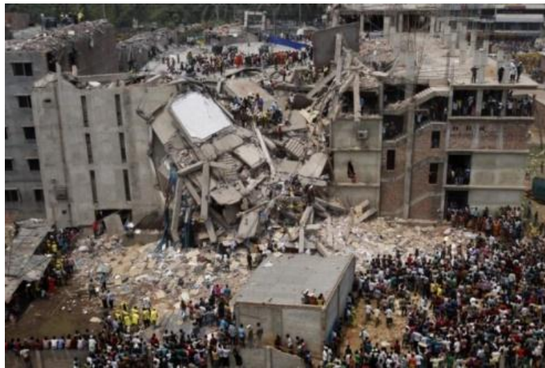
Fig. 3.14. Collapse of the complex Savar, Bangladesh, 2013
