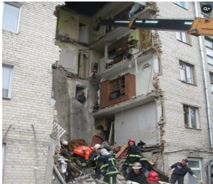
Fig. 3.8. Building collapse, Lutsk, Ukraine, 2012
