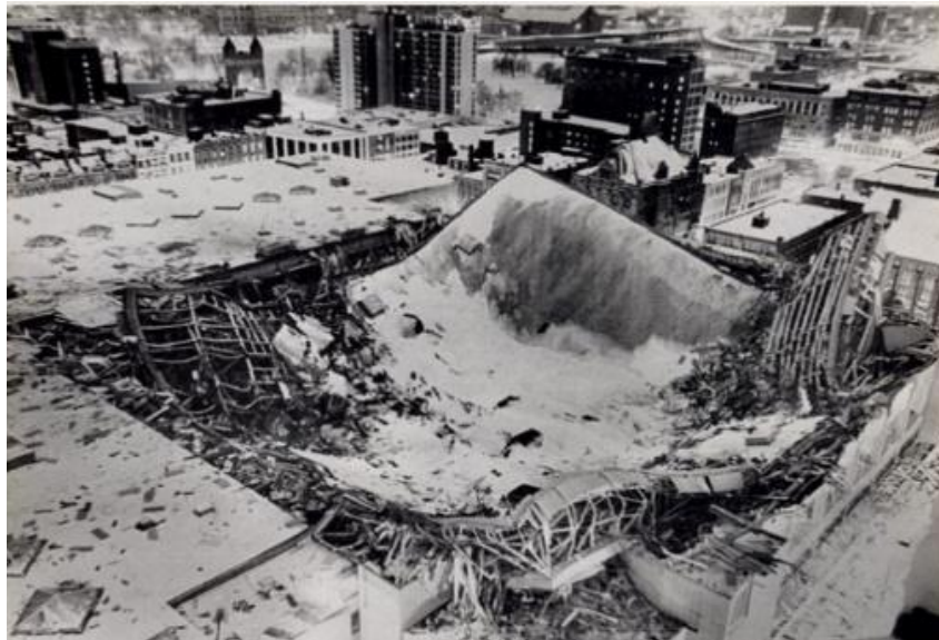
Fig. 3.9. The fall of a sports arena, Hartford, USA, 1978
