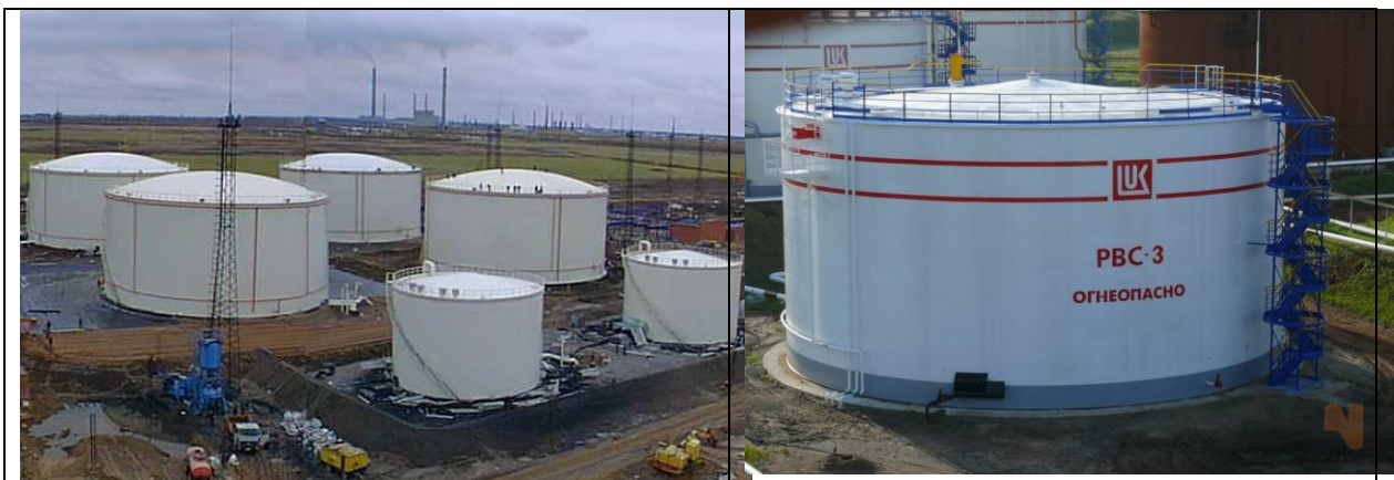
Fig. 11.1. Steel vertical tanks
