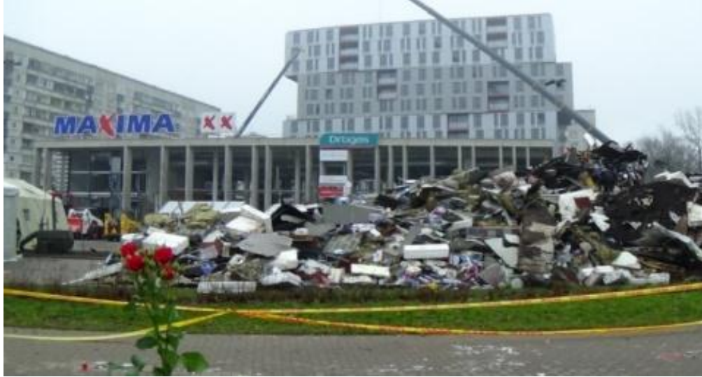
Fig. 3.13. Collapse of the Maxima Shopping Center Riga, Latvia, 2013
