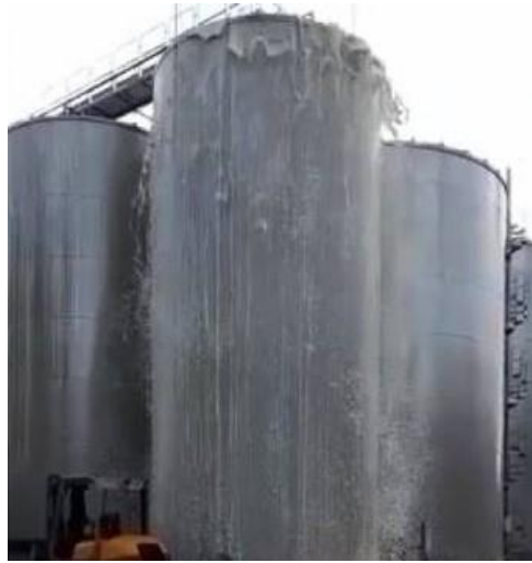
Fig. 11.4. An accident at a winery in Italy, (30 thousand liters of prosecco leaked onto asphalt, 2018)
