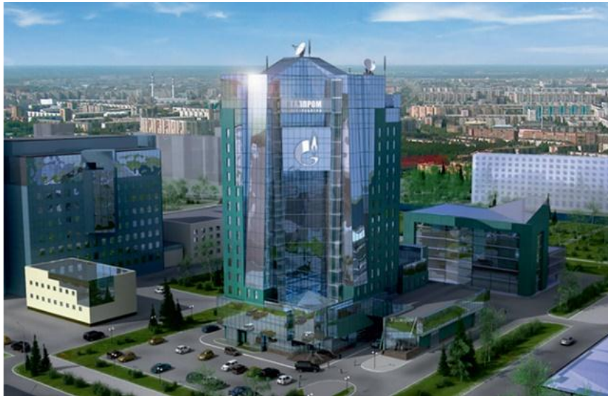
Fig. 3.4. Building project of administrative and domestic office of Gazprom Recycling LLC, in which the flooring collapsed
