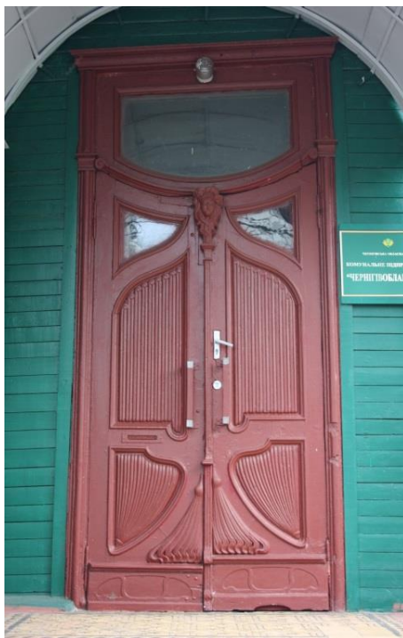
Fig. 6. The front door of the house on the 39 Kotsyubinsky Street
