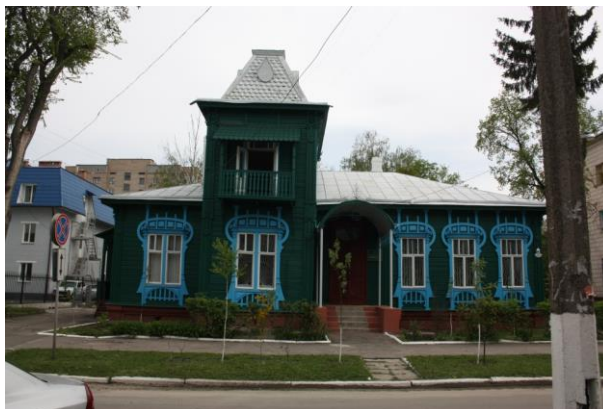
Fig. 3. Building on the 39 Kotsiubynskyi Street
