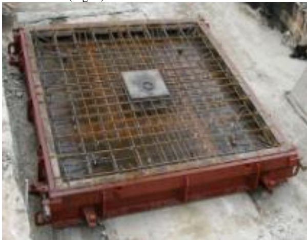
Fig. 5: The location of the reinforcement in the slab formwork
