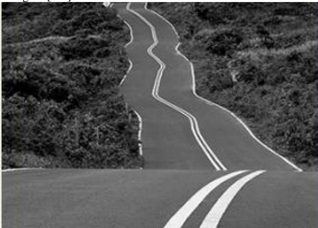
Fig. 1: Example of vertical alignment
