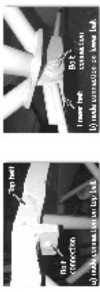
Fig. 2. Node connections of the steel and concrete composite cable space frame
