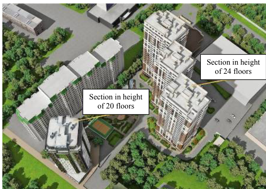
Figure 1 – General view of the residential complex
