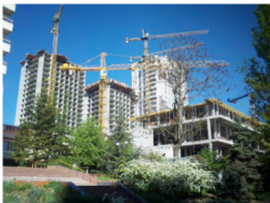
Figure 12 – General view of the frame of sections of the residential complex
