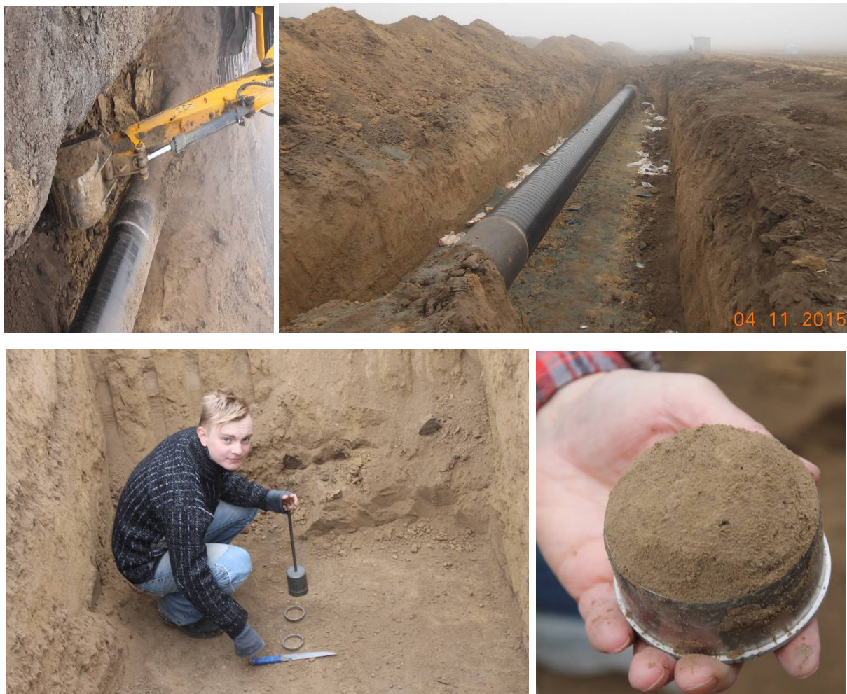
Figure 1 – Loess soil sampling during the pipeline isolation repair works
