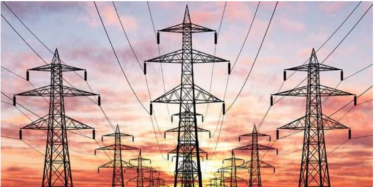
Figure 1.5 - Overhead power lines
