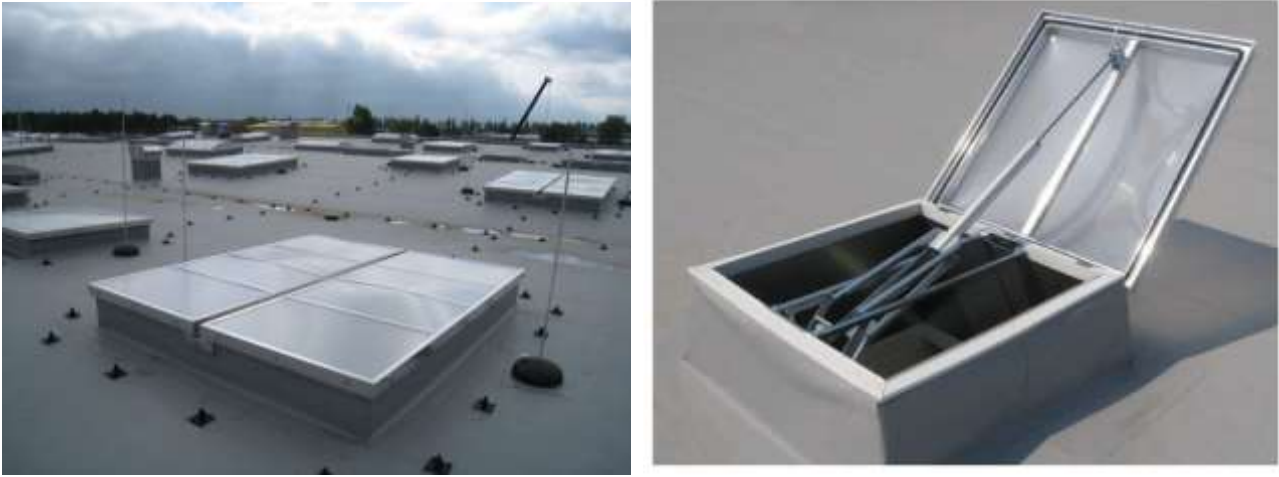
Figure 4 – Photo of placement of anti-aircraft flat lights; the scheme of opening of a lantern for the purpose of smoke removal.
