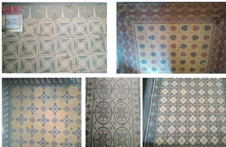
Fig. 3. Ceramic mettlah tiles in the buildings of Ivano-Frankivsk and Kolomyia (identical to mettlah tiles in Lviv).
