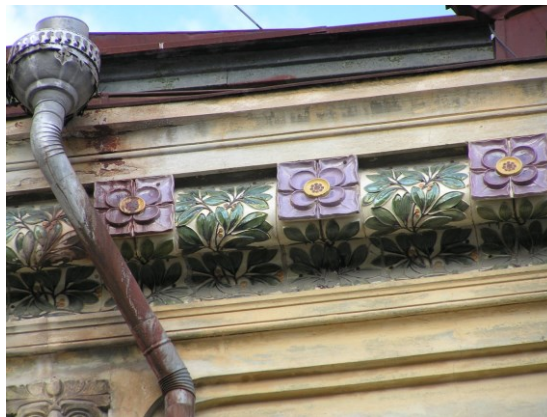
Fig. 9. Ceramic decoration of the facade of the house at 5 Morska Street.
