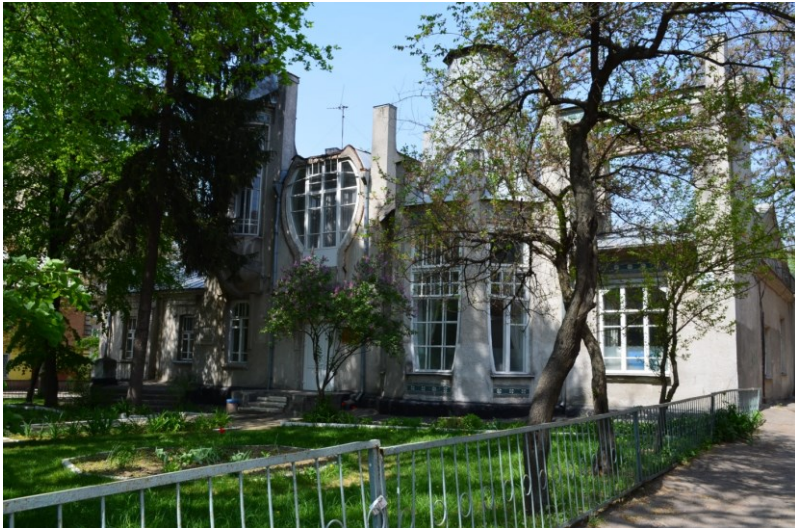
Fig. 4. The mansion of doctor L. Dlugolentskyi in Vinnytsia. General view of the main façade.
