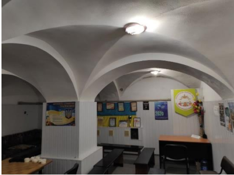
Photo 4. Cross vaulted ceiling in the basement of the Land Bank Building
