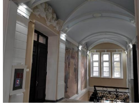
Photo 5. The cross vault in the Land Bank Building
