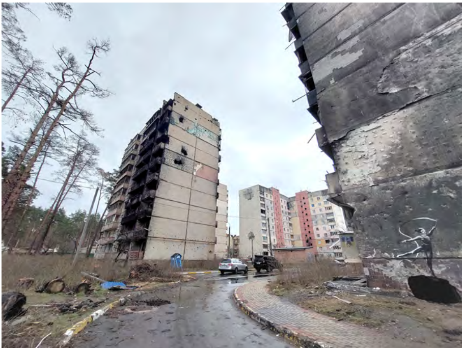
Fig. 10. Destroyed residential buildings in Borodianka (photo: Yulia Ivashko)
