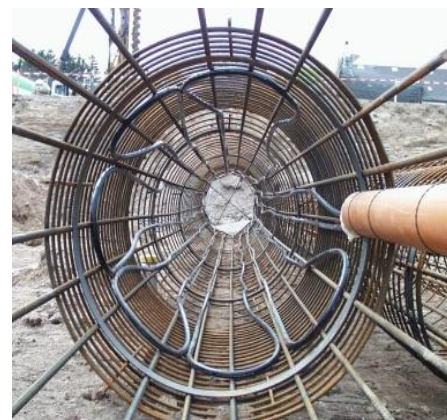
Figure 3. Energy pile
