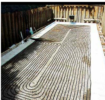
Figure 2. Laying pipes under the foundation slab
