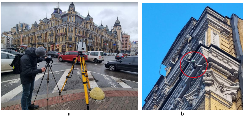
Fig. 3. The process of visual inspection of the building (photo by Oleksandr Molodid, 2021): a – photographing the building in parallel with the creation of its 3D model; b - photographing hard-to-reach places with the involvement of a drone
