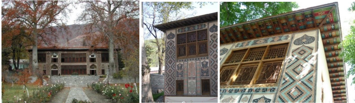
Fig.1. Palace of Sheki khans. General view and details of façade ornamentation
