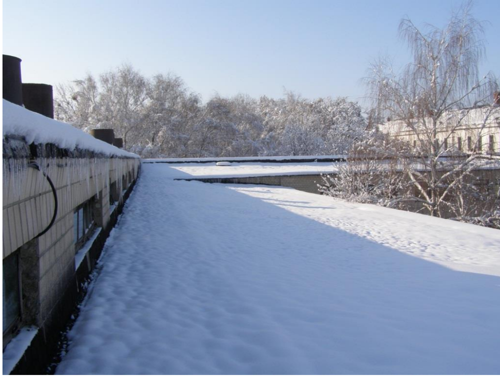
Fig. 10.7. Snow cover on the fuel roof
