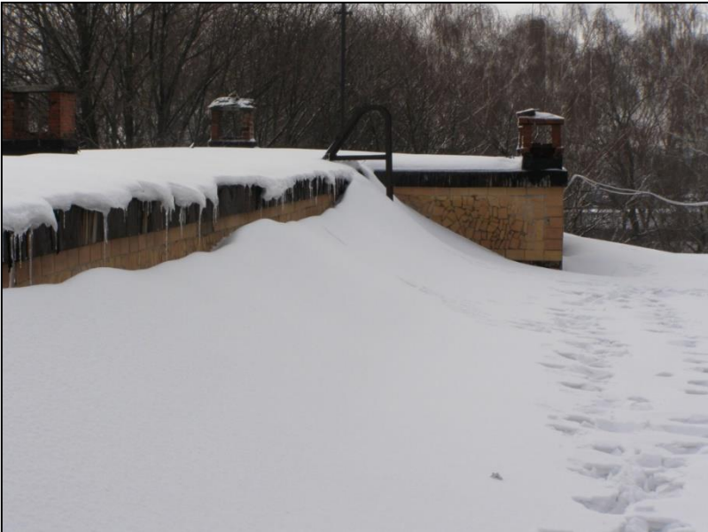
Fig.10.11. Snow deposition at roof height differences (snow bags)
